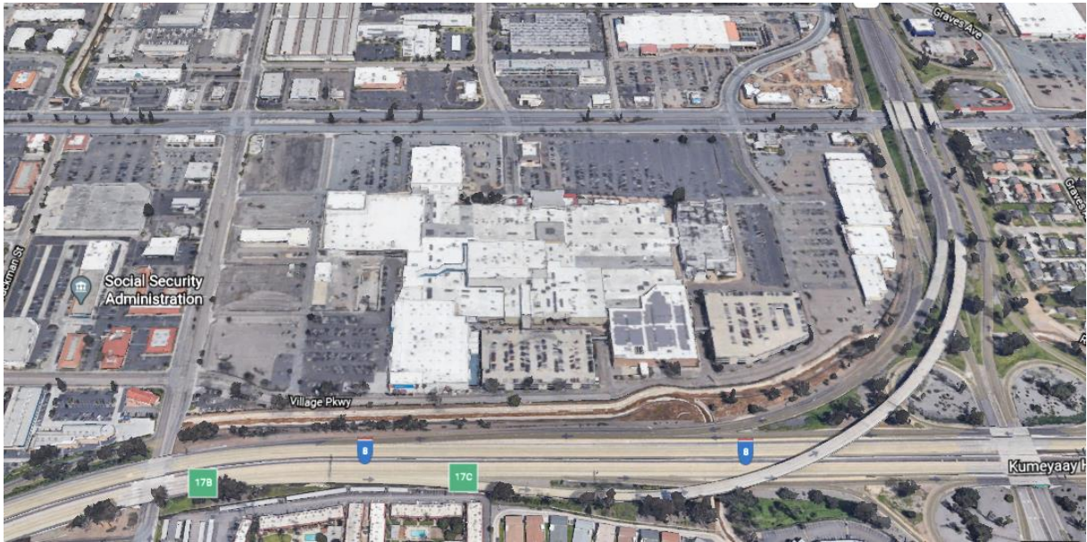
Figure 1. Parkway Plaza, El Cajon (Google Earth Image, facing North, retrieved 5/20/2022 from: https://earth.google.com/web/search/415+Parkway+Plaza,+El+Cajon,+CA )
