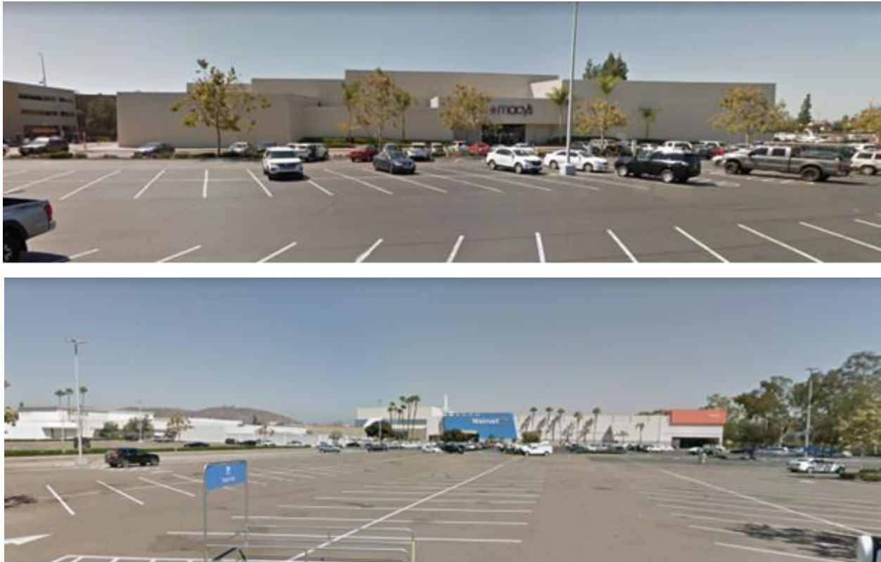
Figure 2. Site Photos: Parkway Plaza, facing Macy's and Walmart's from Parking Lot (Google Earth, 2022)
